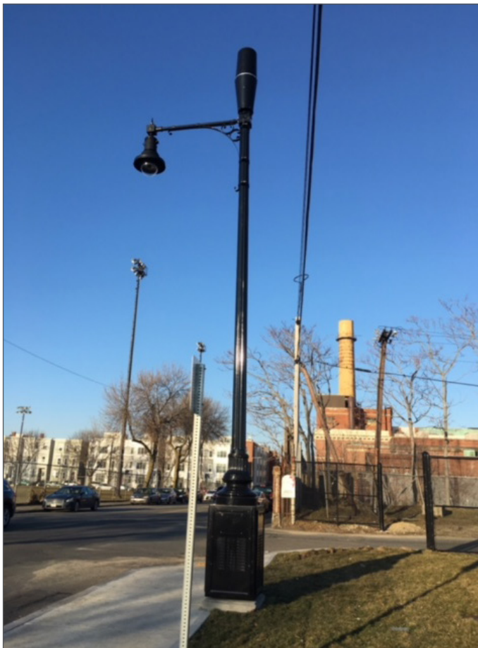
Figure 4.20-G Small Cell Node Allowed Configuration
